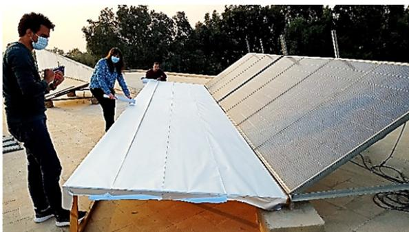
Fig.24 Fixing stage of the reflectors
