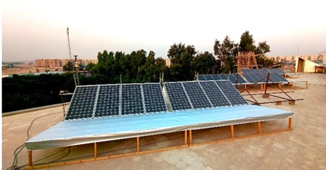
Fig.25 Final stage of the reflectors
